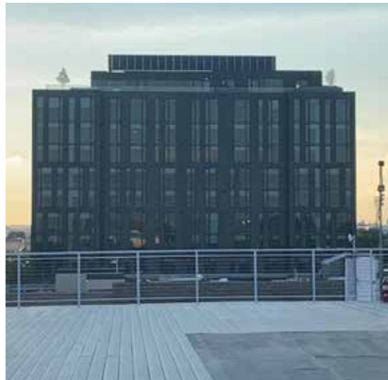
Sample photo of vertical panels, Union Market, DC
